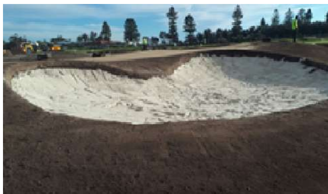
Shaping the practice bunker
