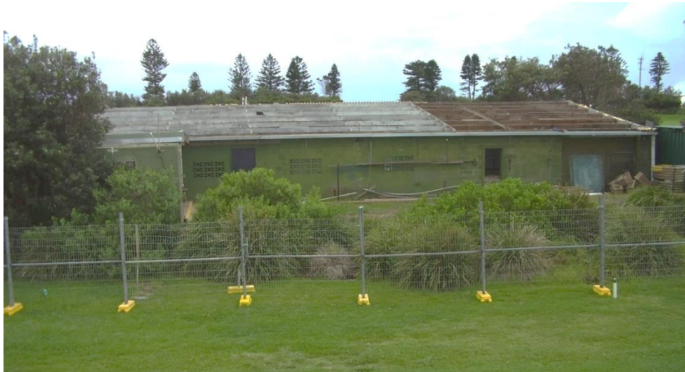
Demolition of the old, 1970's Green keeper's shed
