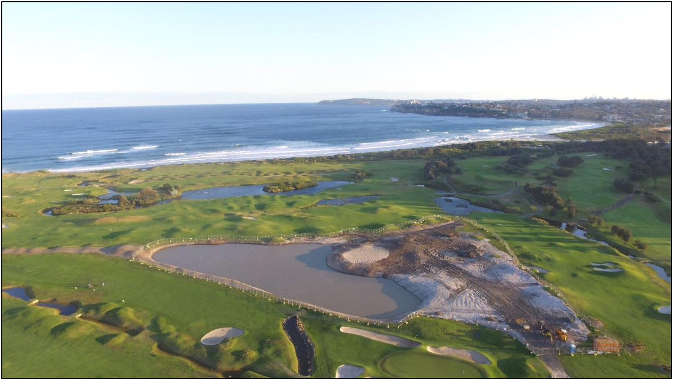
Construction of dam completing the wetlands project, 2019
